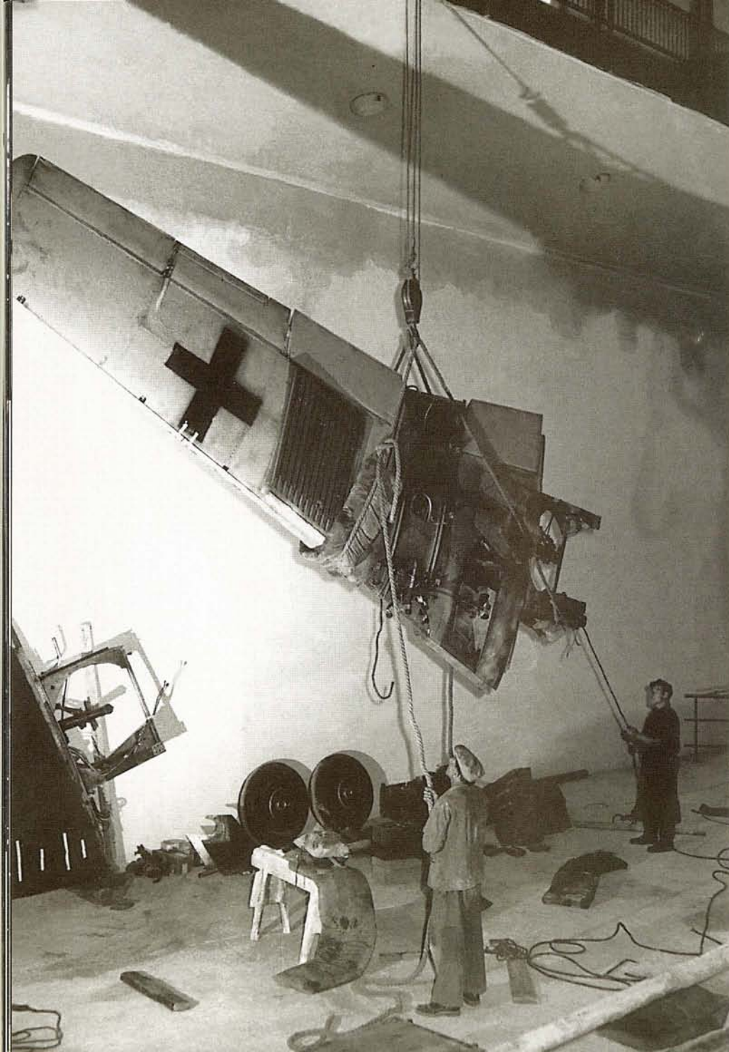
▲ Employees of the Deutsches Museum give an impression of the size of the Me 262 wing. The surfaces between the wing root and the engine nacelles had not been painted, as is evident in this view. The wing was attached to the fuselage by two 20 mm (0.78 In) and forty-two 8 mm (0.3 In) bolts at four points. During the transport from Dübendorf, Switzerland, to Munich, the main wheel leg remained in the main wheel well. (Deutsches Museum München)
